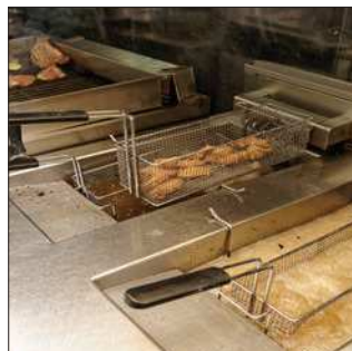
Grease Waste Flow Maintenance
